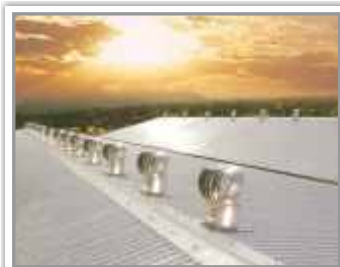
Rooftop Wind Ventilator
